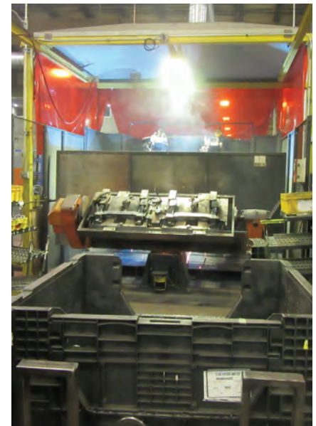
ATLANTA — A robotic prototype welding on a postioner.
