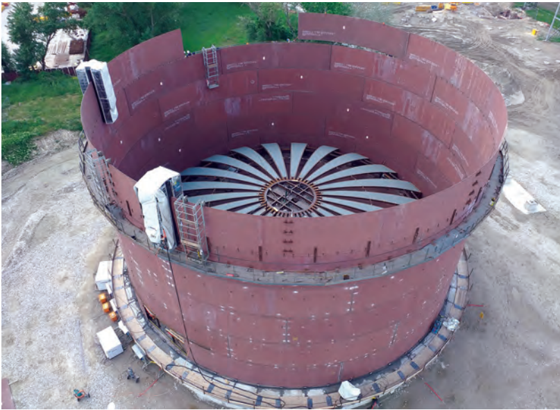
Fig. 5 — Setting up the final ring of a LNG tank for DSAW.
